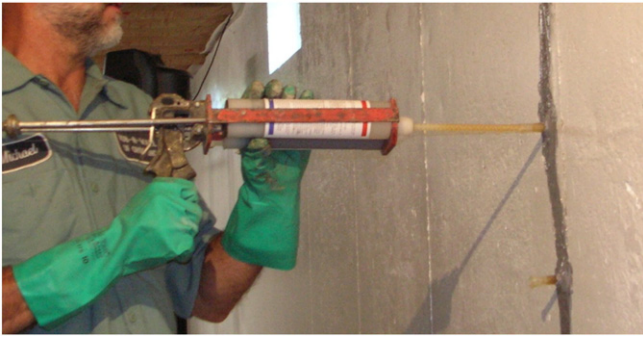
Fig. 1. Conventional manual procedure of fissure injection.
