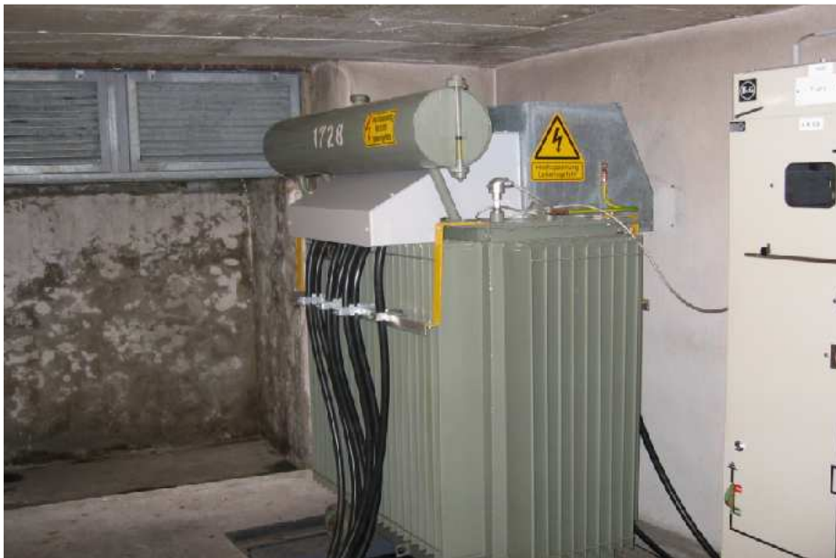
Figure 33: “MV/LV TRANSFORMER”
