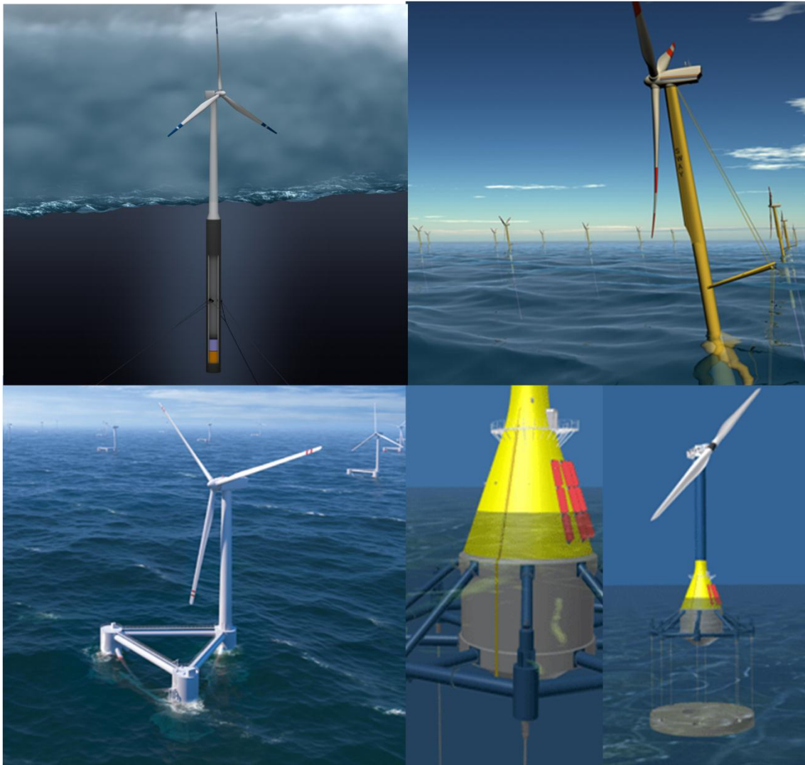
Figure 7. Floating support structures Hywind (spar) - Sway (spar) - WindFloat (semisubmersible) - Blue H (TLP) [44 - 45 - 46 - 47]
