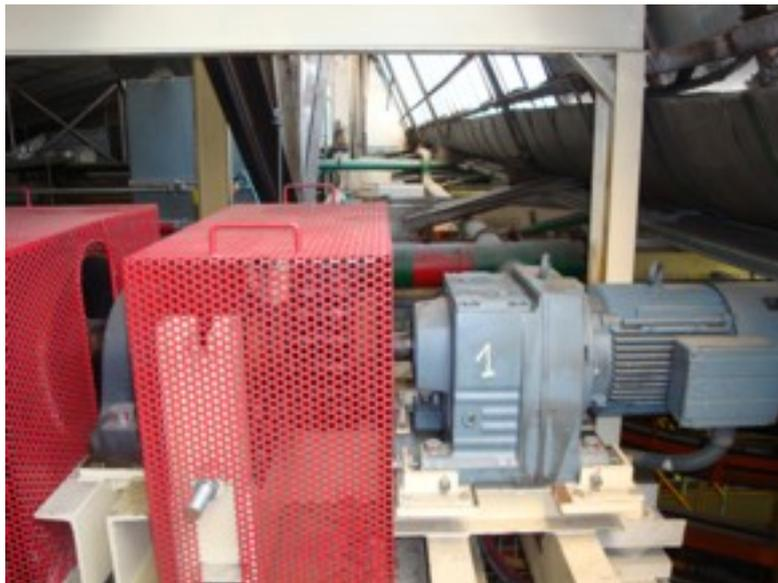
*Figura 4.15. Motor reductor principal*
