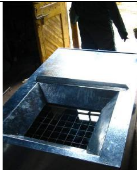
Finally the cover is placed on the box and is riveted.
